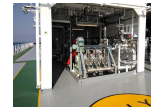
More than 40 diaphragm process pumps installed on vessels for LPG FGSS
